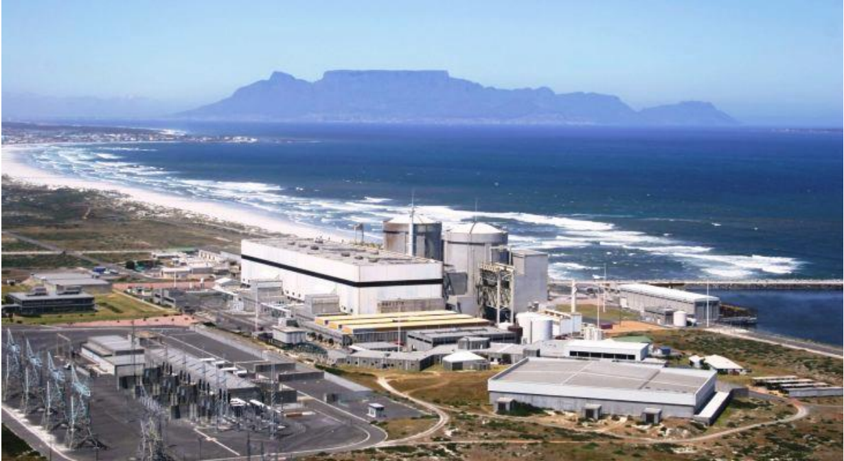
Figure 16 Koeberg Nuclear Power Plant
