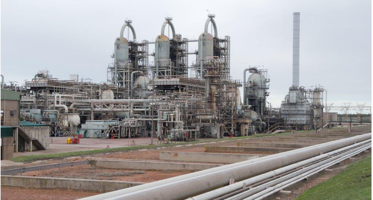
Figure 13 PetroSA gas to liquids facility in Mossel Bay, Western Cape
