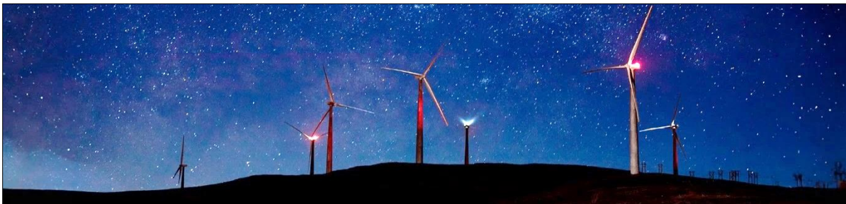
Figure 8 Red Rocket Energy wind turbines (Roggeveld, Western Cape)
