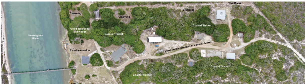
AERIAL PHOTO OF EXISTING BUILT AREA AT PORTION 4
